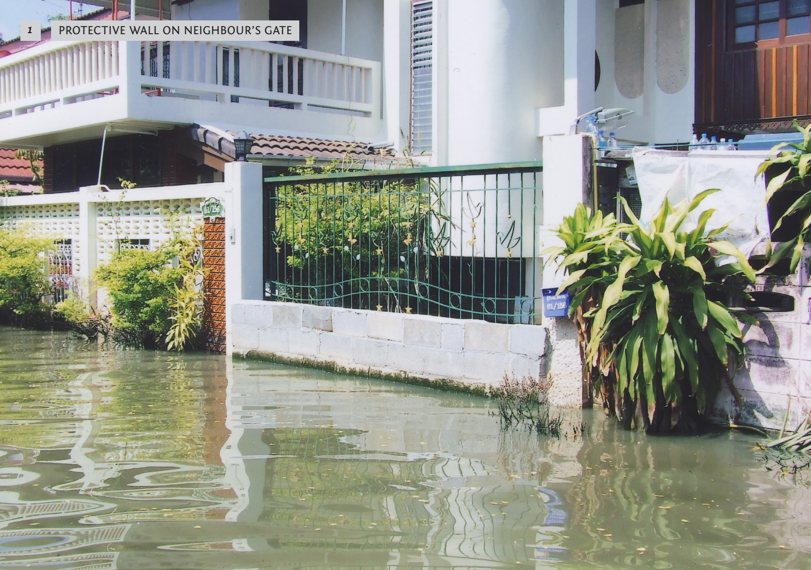
2 SANDBAGS AT NEIGHBOUR'S GATE
